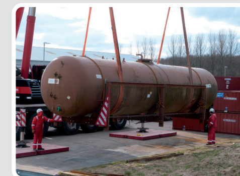
Unloading of large oil tank at the Studsvik MRF
