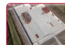
View of vault 9
