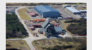
LLWR Grouting Facility
