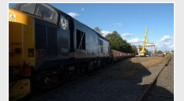
Containers being delivered by rail
